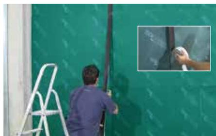
When all panels are fixed seal the panel joints with the Stik tape. Build the second wall.
