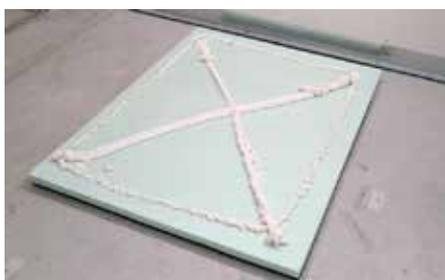
Or apply the glue Selena Tytan's on the panel laid on the ground.
