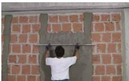
Apply in the first wall a layer of row mortar of about 1 cm thickness.
