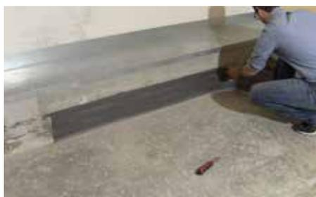
Clean the floor area and apply the Profyle Flat edging strip vertically, around the perimeter of the room
