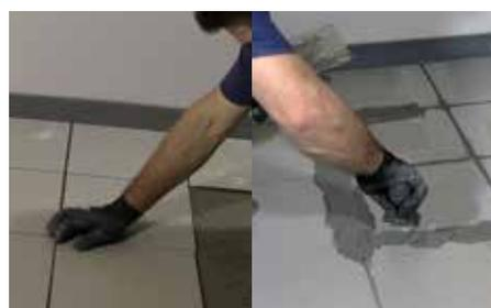
Lay the tiles on the adhesive, as desired. Apply the grout and clean the ceramic tiles
