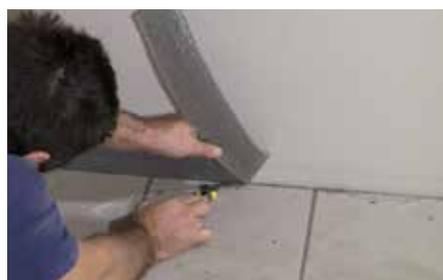
Trim the Profyle edging strips, only when the floor finish has been completely installed
