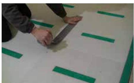
Seal any gap between two adjacent components with Stik tape
