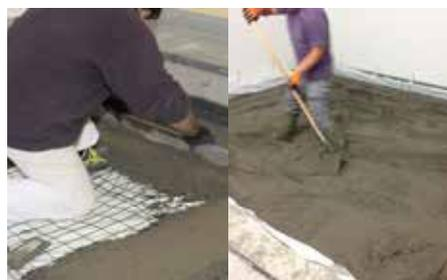
Build the screed (sand and cement or self-levelling), reinforced with reinforcement mesh
