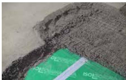
Build the screed, if necessary reinforce the screed with a steel mesh
