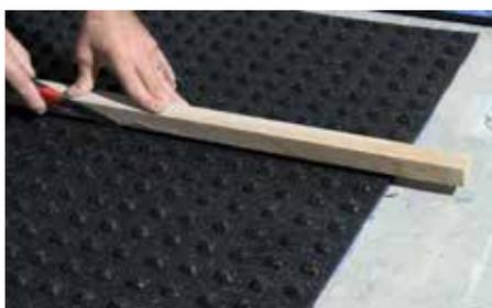
Where necessary, cut the panels with a sharp knife
