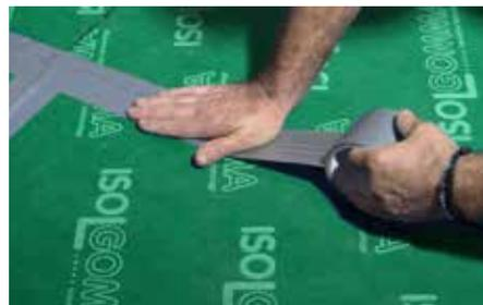
Seal the joints between panels with Stik tape
