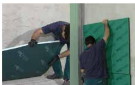
Apply the panel on the wall by forcing with homogeneous pressure.
