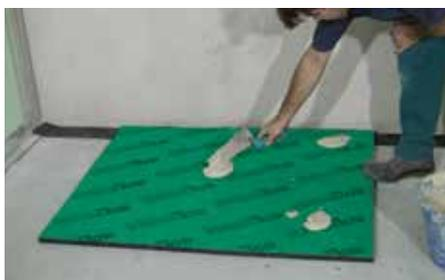
Apply the glue on the panel in dots (5 dots per panel).
