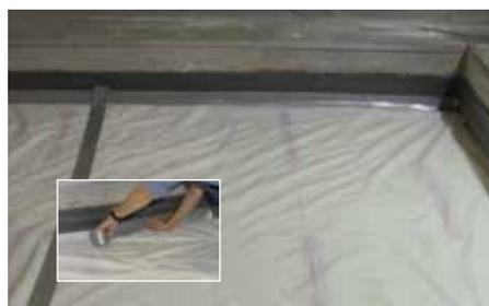
Place a protective layer/film. Protecting precisely the surface sides and junctions with stick
