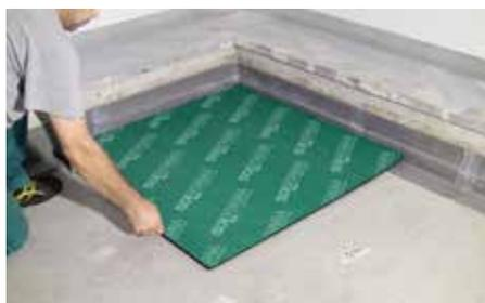
Install the acoustic mat with dimpled side facing down
